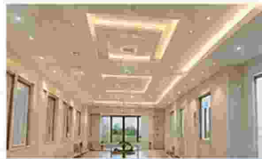
GYPSUM CEILING WORKS
