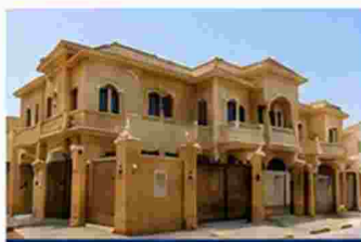
VILLA RENOVATION – AIN KHALED
