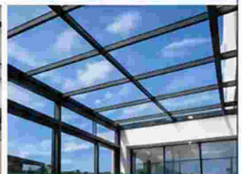
SKYLIGHT & ROOF GLAZING
