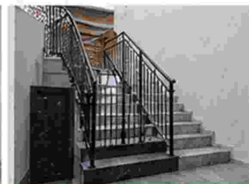
STEEL HANDRAIL WORKS
