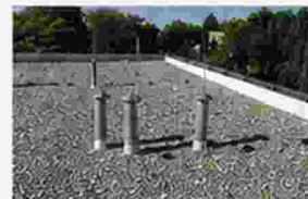
GRAVEL ROOF WATERPROOFING
