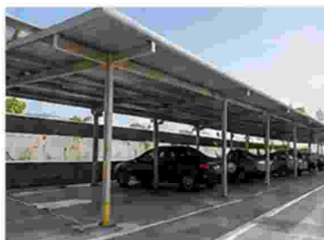
CAR PARK SHED
