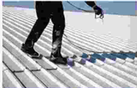
METAL ROOF WATERPROOFING
